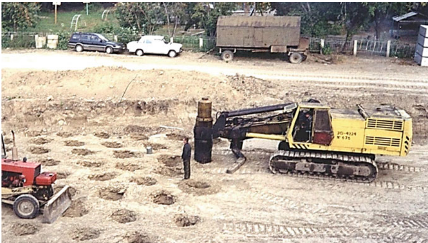
Fig. 1 Unit for deep soil compaction
